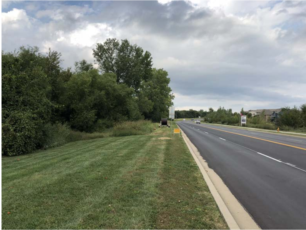
View looking north from south property line
