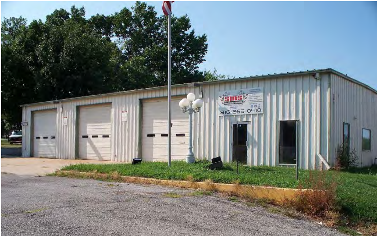
View looking from 58 Highway
