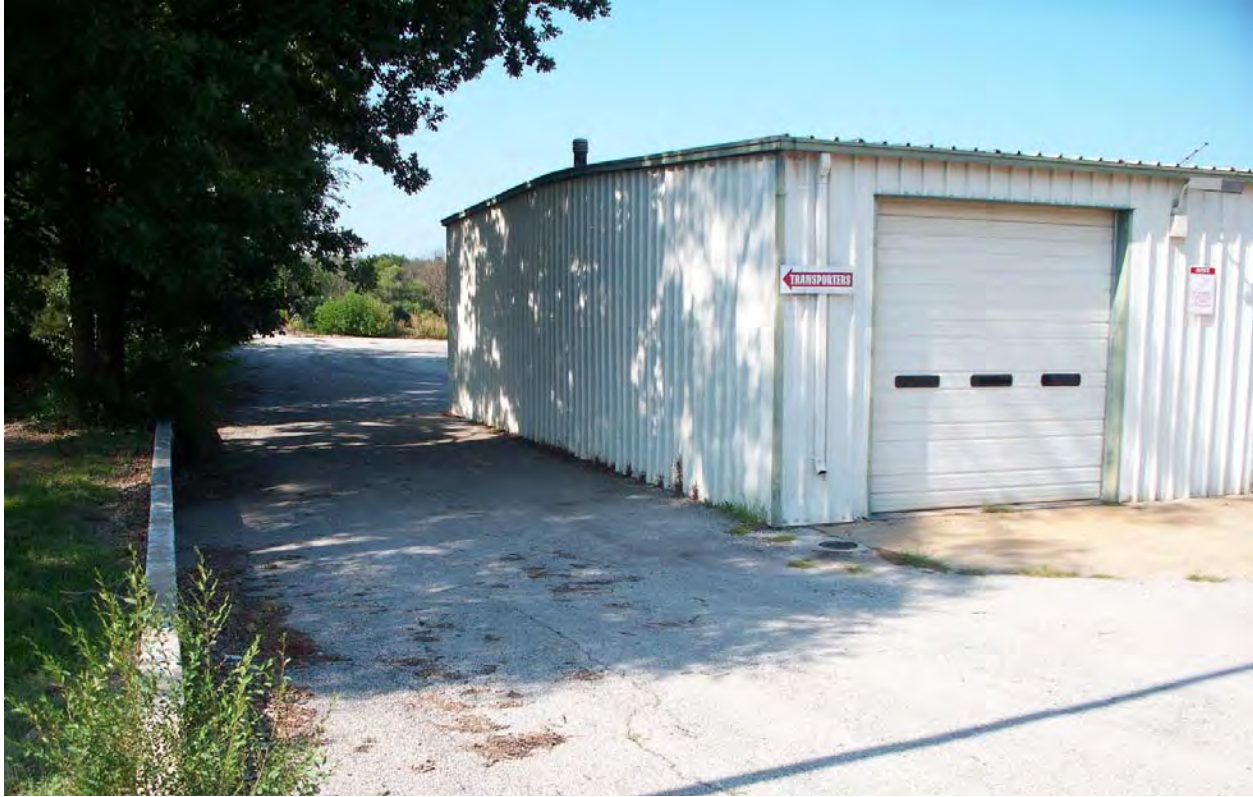
View looking north along the access drive from 58 Highway
