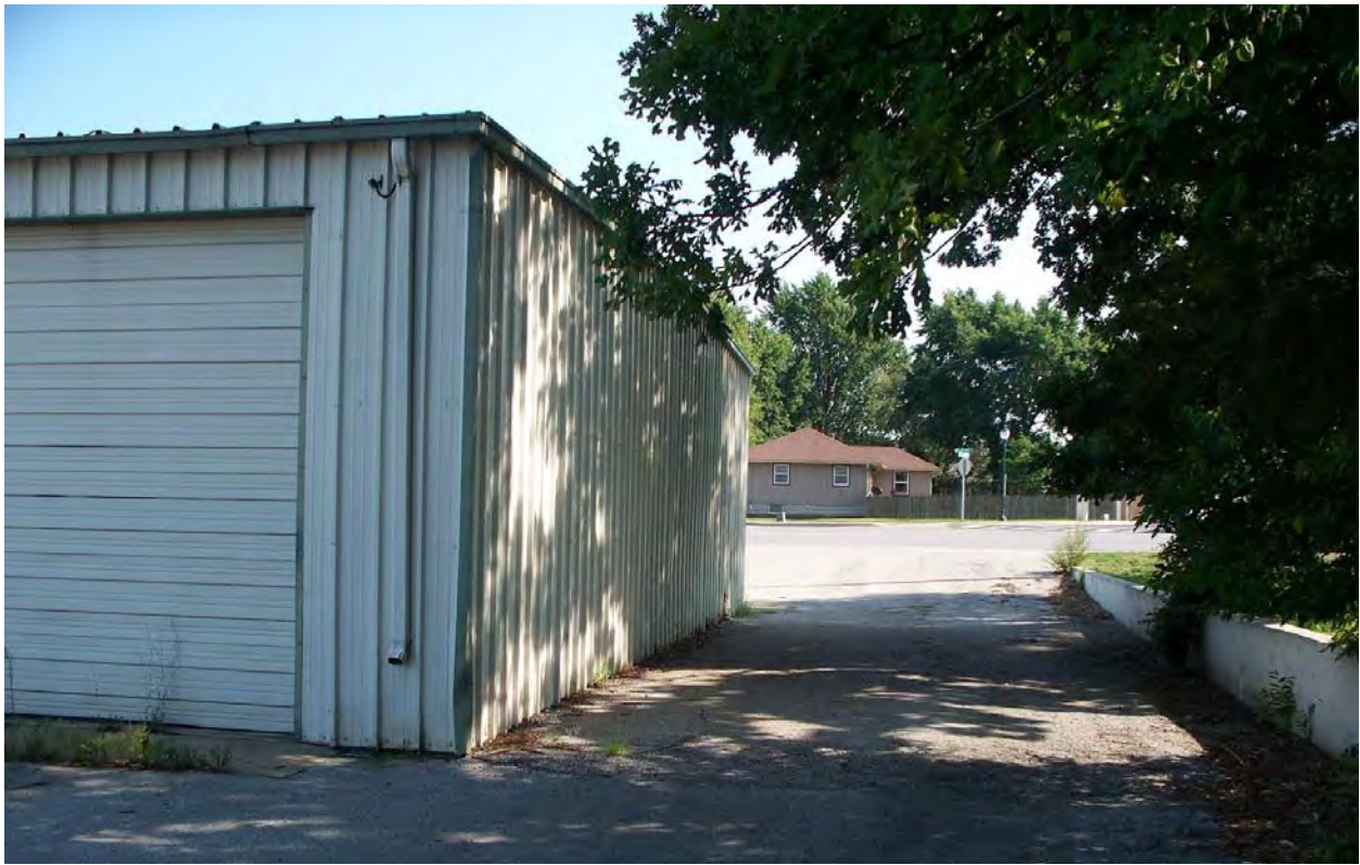
View looking south along the access drive from 58 Highway.
