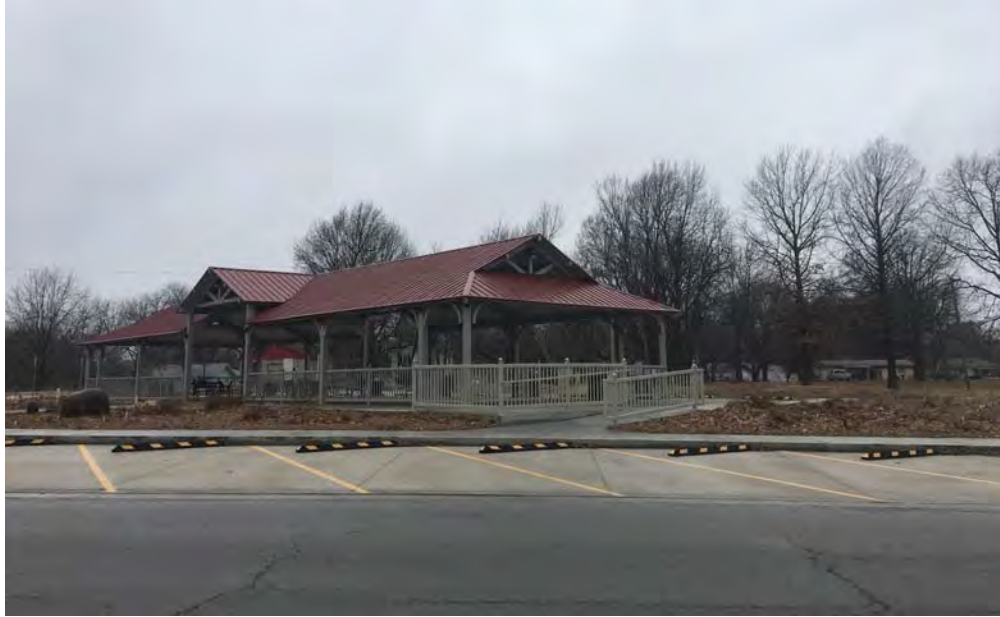
View looking west showing the angled parking along S. Washington Street
