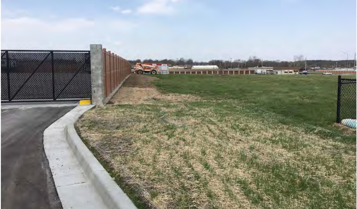
(View looking east along the southern property line)
