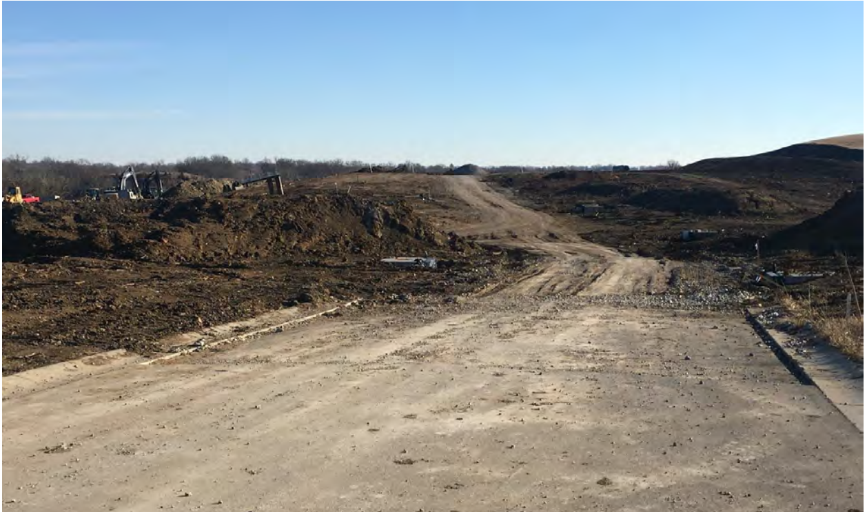
(View looking south from Bridgshire Drive)
