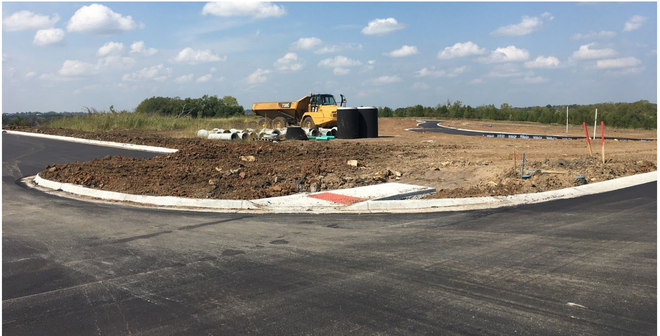
(View from Granshire Lane and Bentwater Drive looking northeast)
