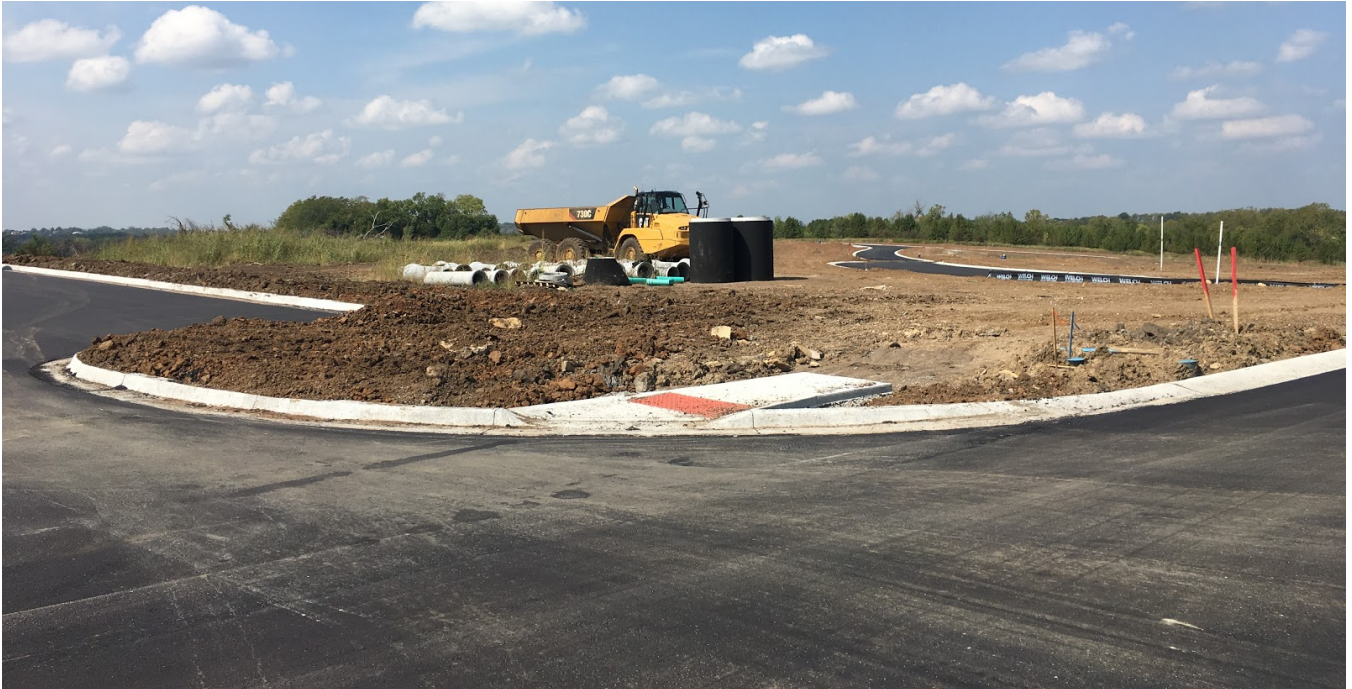
(View from Granshire Lane and Bentwater Drive looking northeast)
