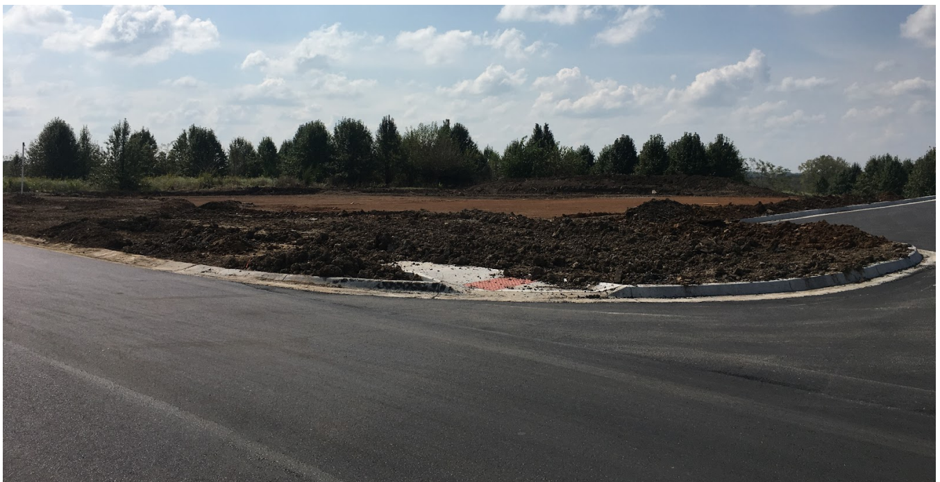
(View from Granshire Lane and Bentwater Drive looking southwest)
