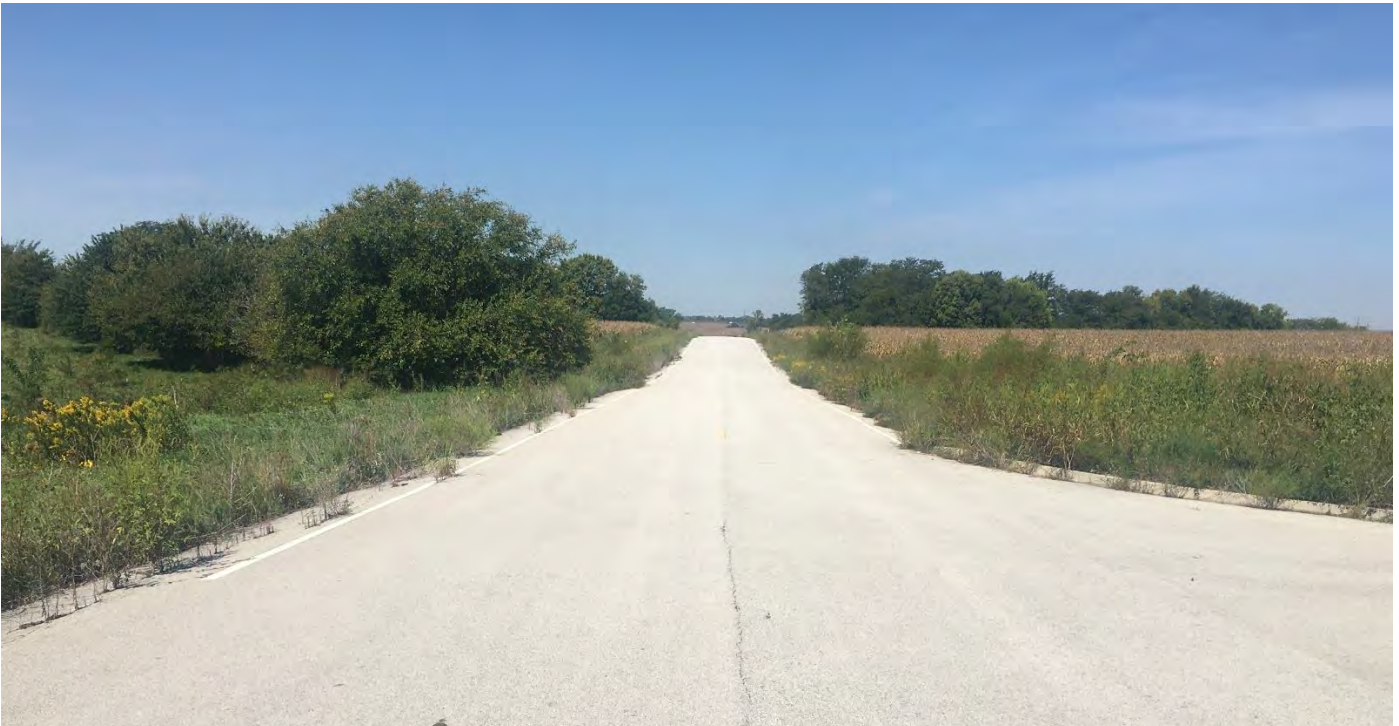
View looking northwest along North Cass Parkway.
