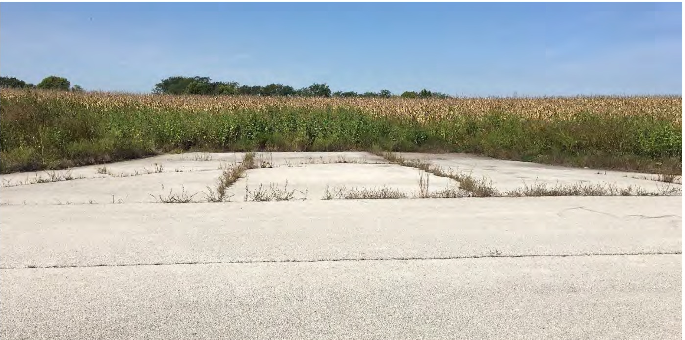
View looking west at the future extension/connection of Forbes Drive from Brook Parkway.
