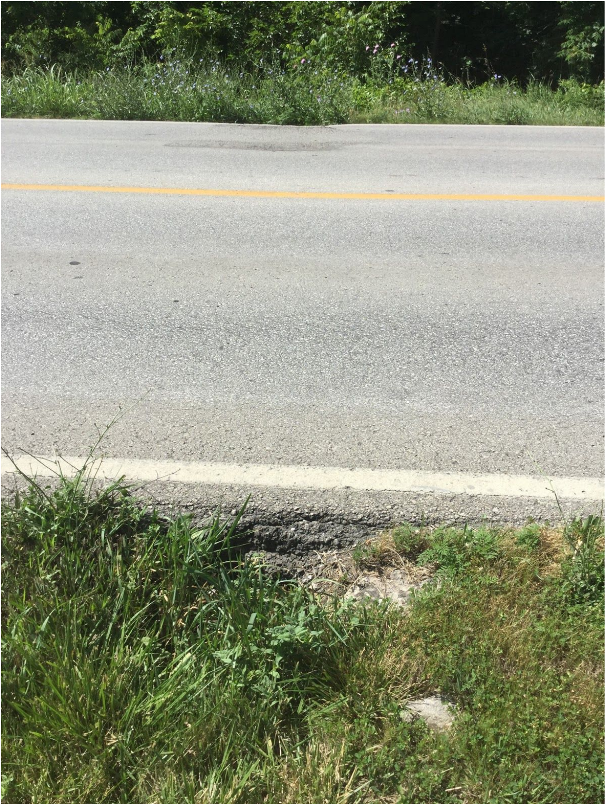
Headwall Repair - Photo #2
