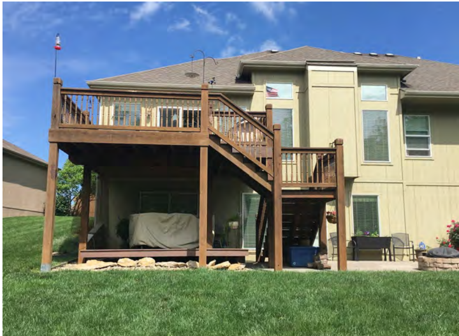
View of the existing deck at 411 S. Fox Ridge Drive
