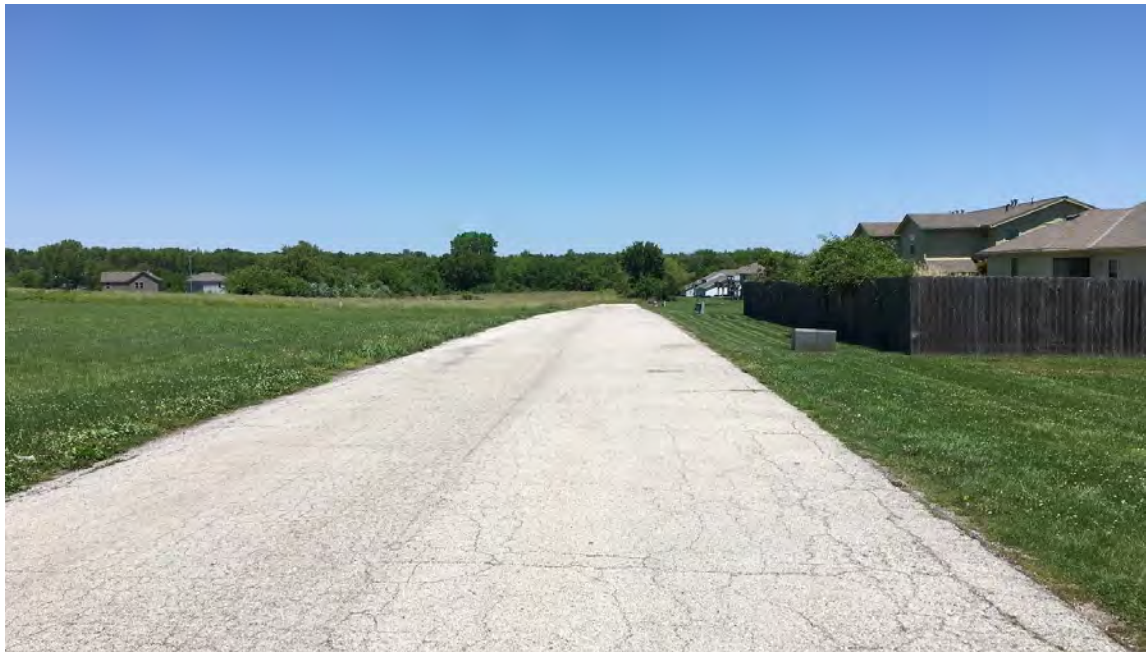
View looking north along the access drive from E. Walnut Street
