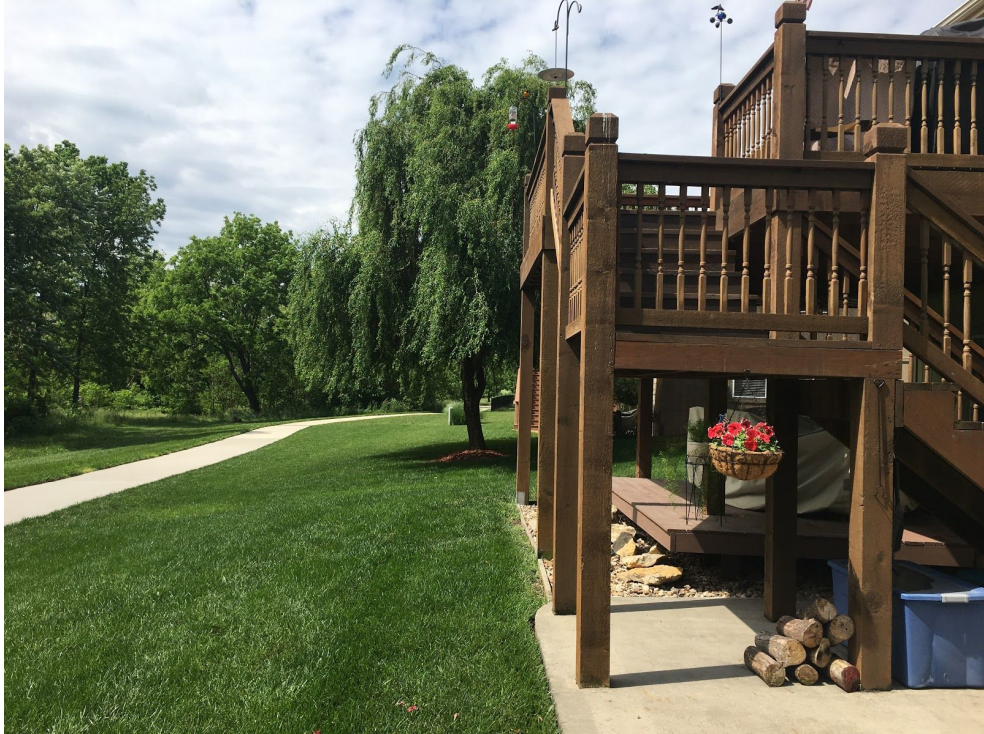
View looking southwest near the rear property line
