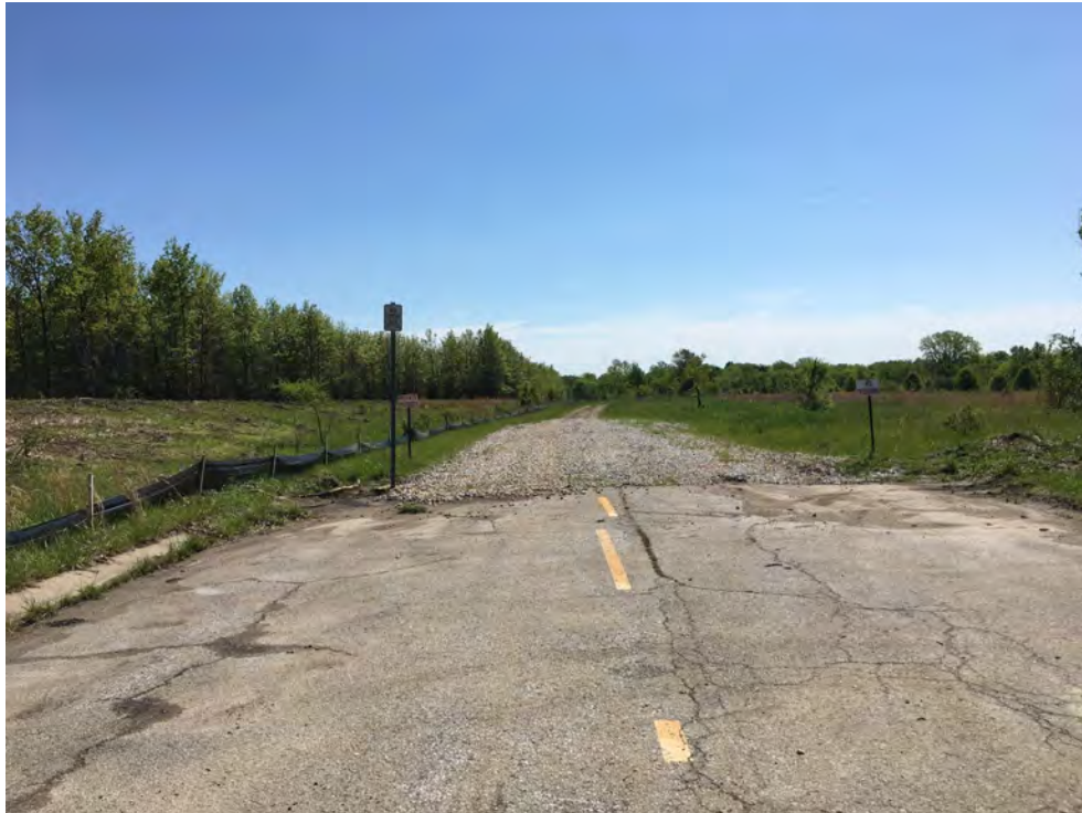
View looking east along Pine Street.
