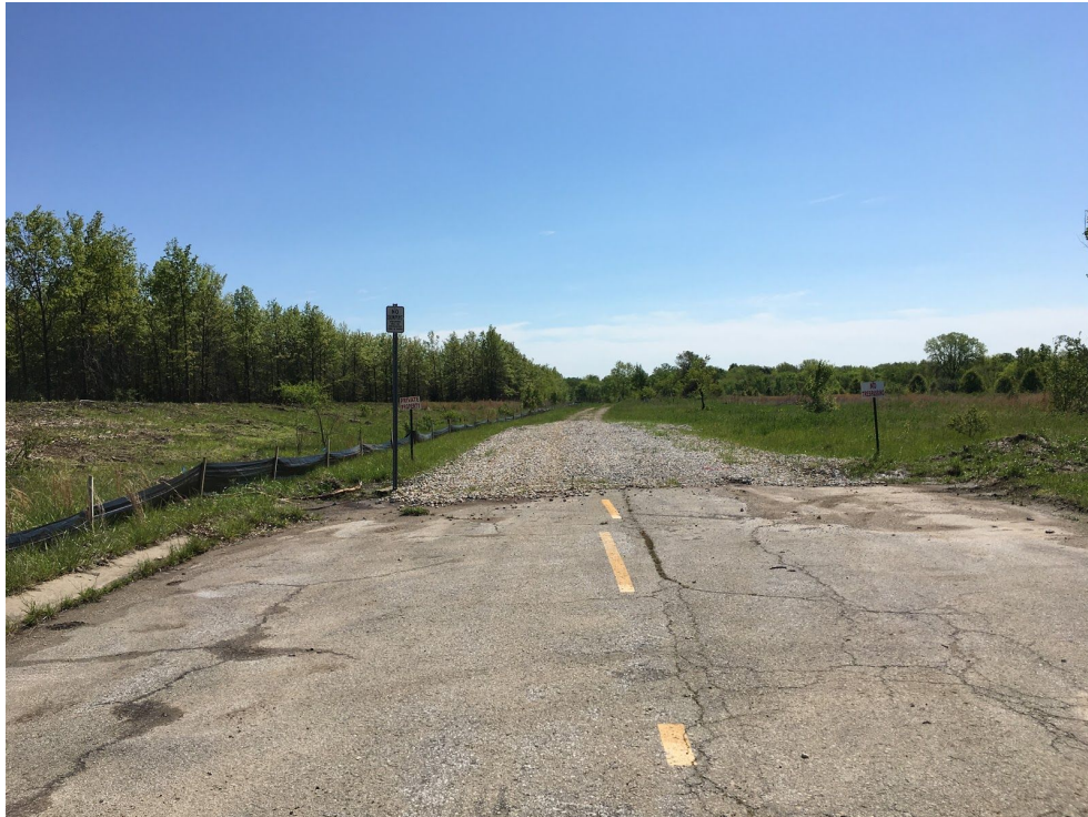
View looking east along Pine Street.
