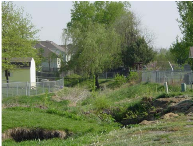
Impacted Second Order Stream in Canter Ridge with Bank Erosion (H)
