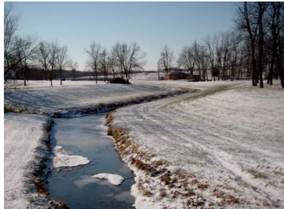
Channelized Trapezoidal Fifth Order Stream at 162nd and Valentine Rd
