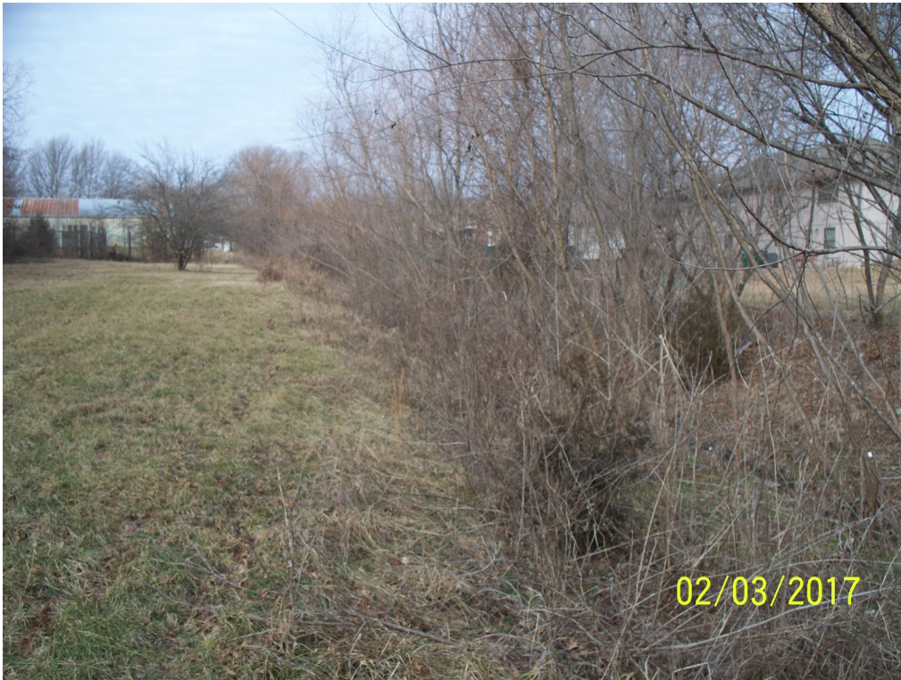
View looking west from Washington Street at drainage swale along north property line
