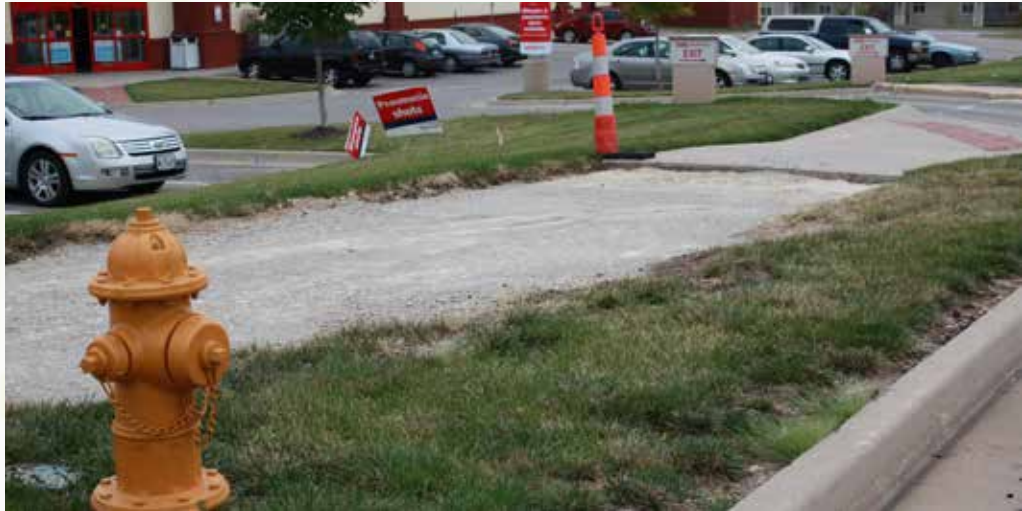
Foxridge Trail south of 58 Hwy under re-construction using new City standard.
