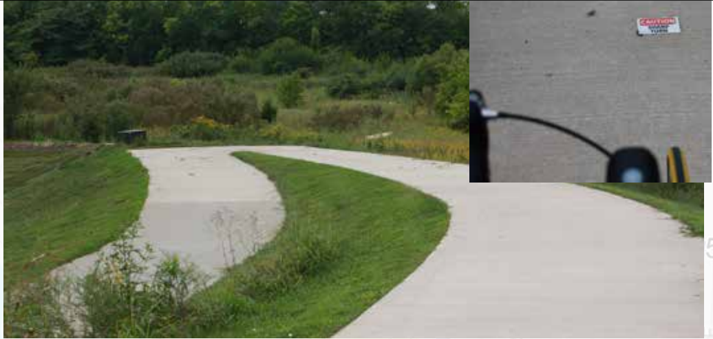
Switchback warning is small sign attached to pavement. Recommend: larger, upright warning signage.
