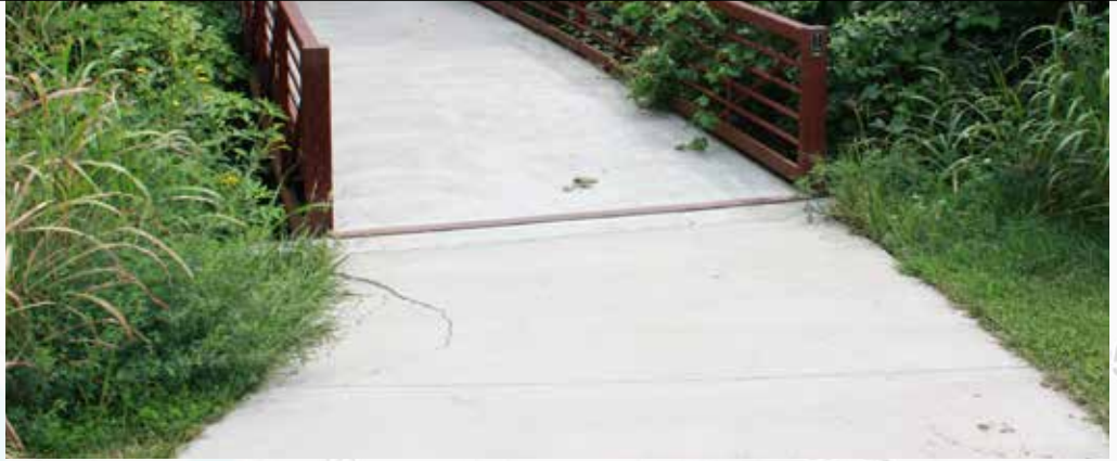
A crack in the walk at bridge abutment. Already identified by Parks Dept. as a winter project. No guard railing present at bridge ends. Recommendation: 45° winged rails for all bridges.
