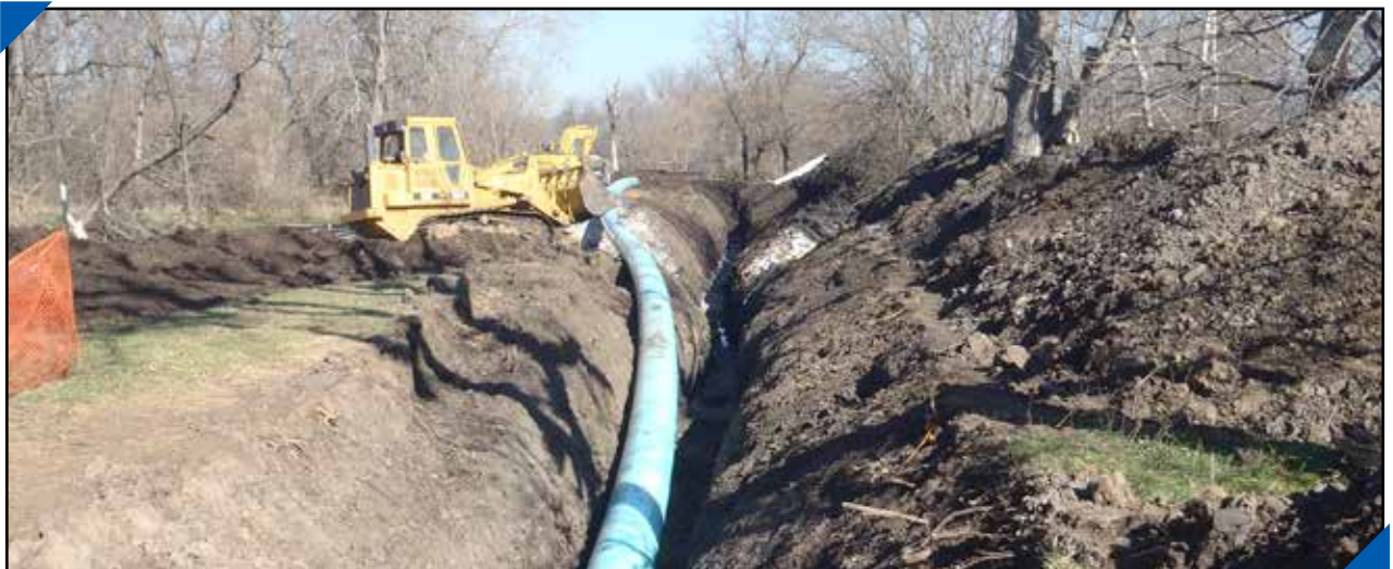
Installation of 24" Replacement Owen Good Force Main
