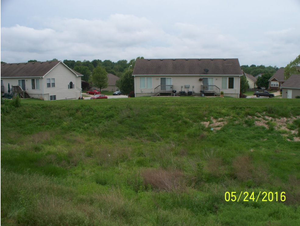
View of Common Area Tract A looking south
