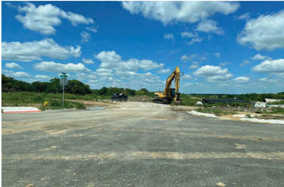
View looking north from 163rd St.
