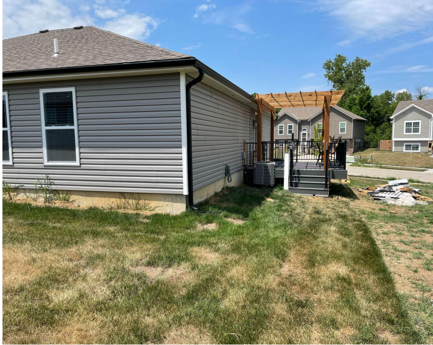
View looking north from southeast corner of subject property
