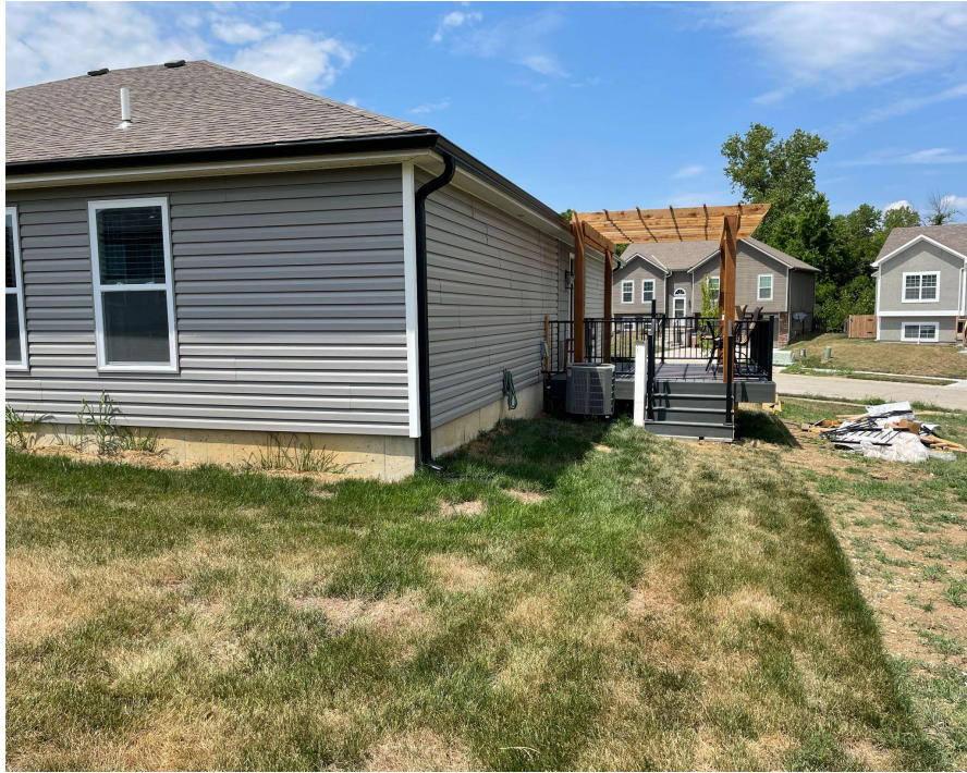
View looking north from southeast corner of subject property
