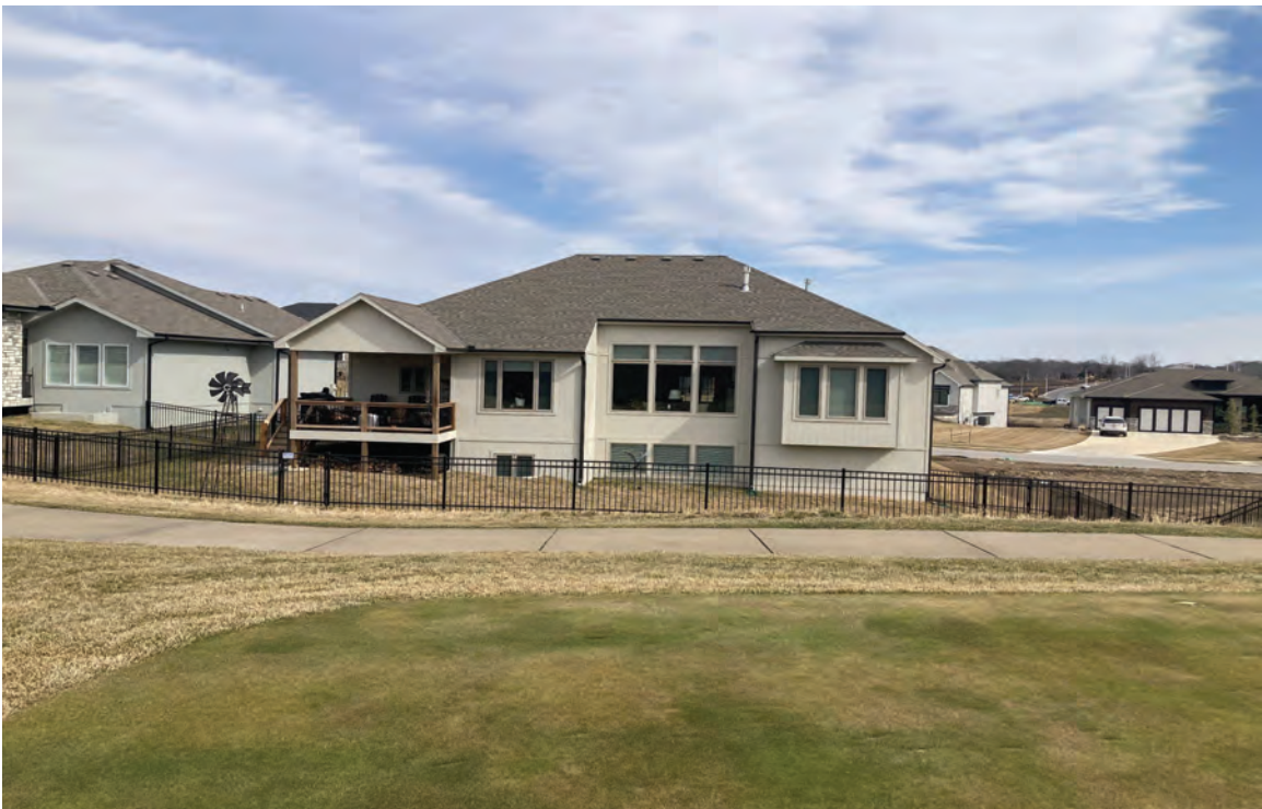
View looking east from west property line
