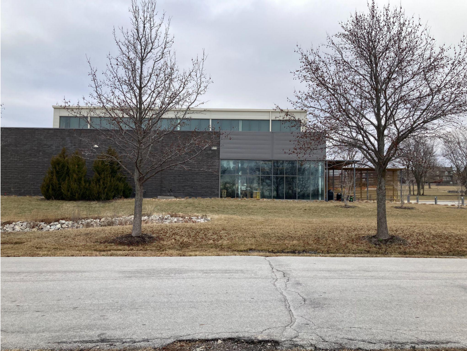
View looking north from primary access road into Recreation Park
