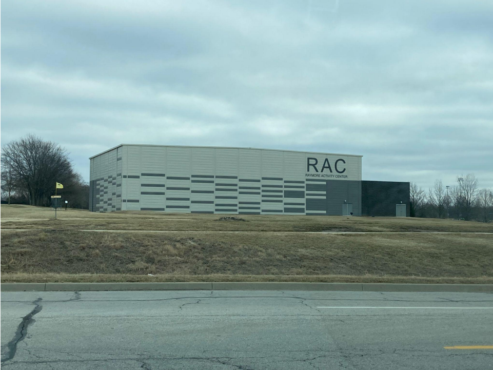
View looking east from S. Madison St.
