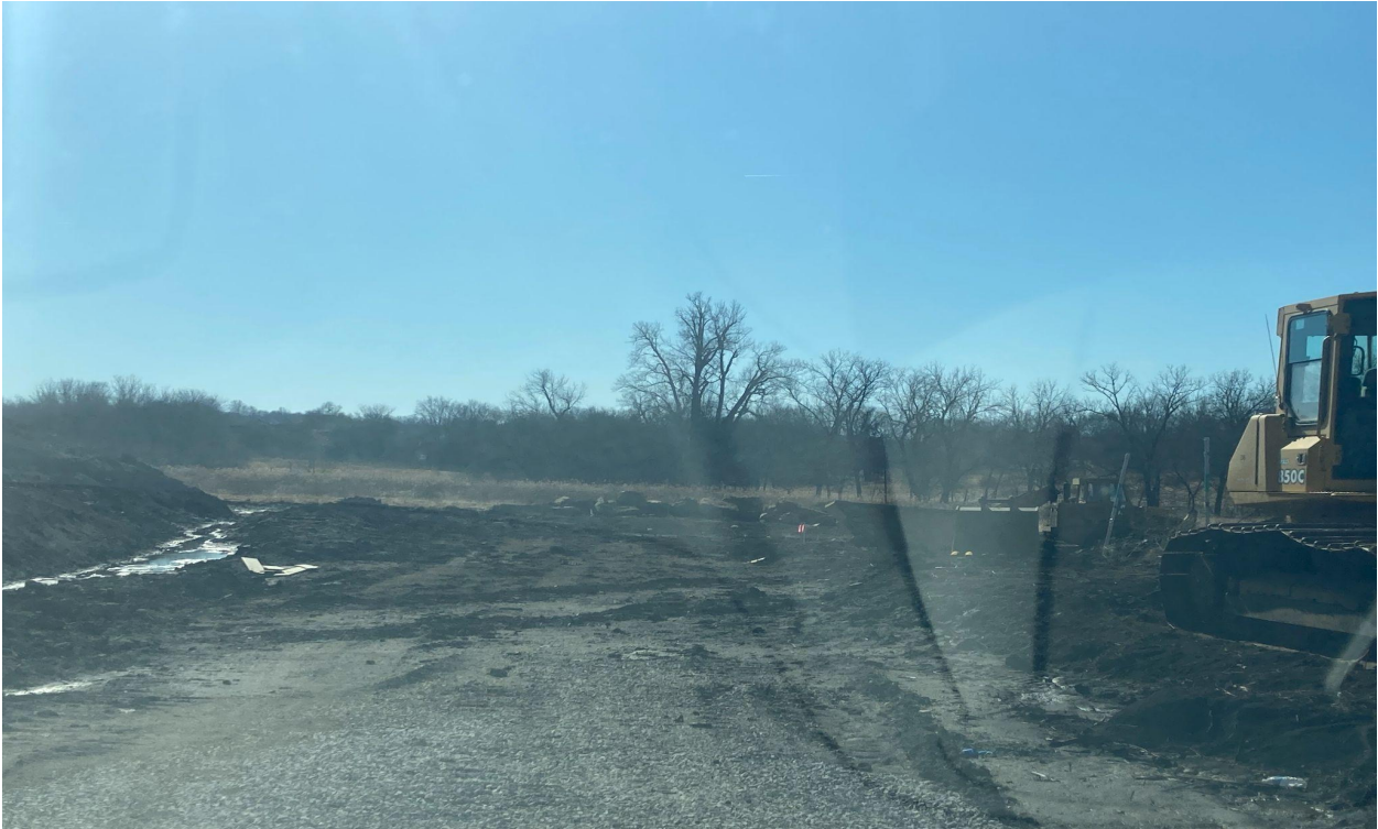
View looking south from existing Eastbrook 3rd Plat (Branchwood Ln.)
