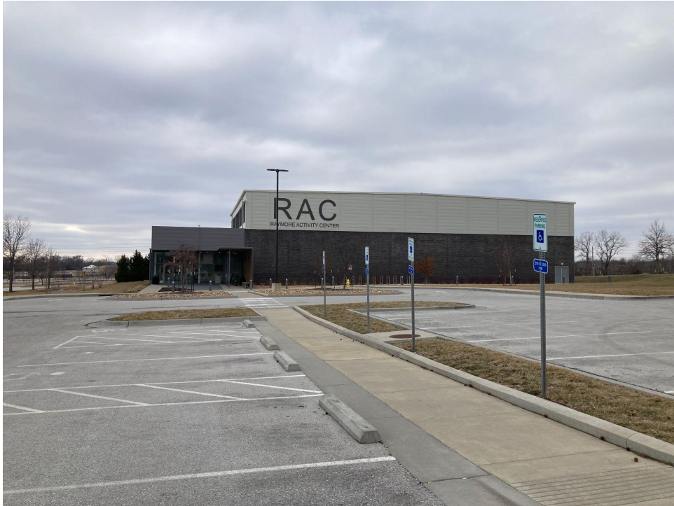
View looking west from existing parking lot
