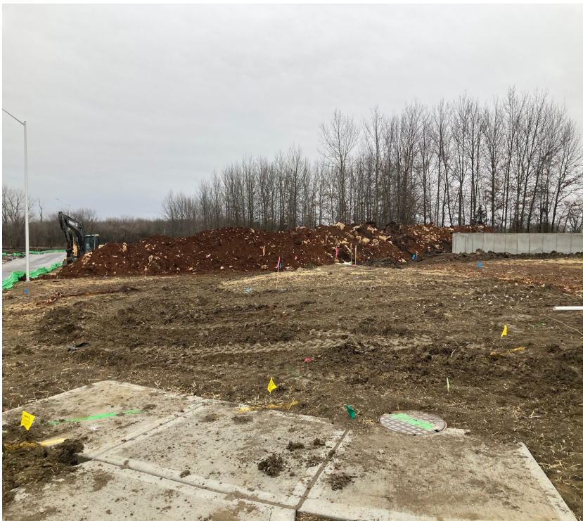
View looking east from N. Franklin St.
