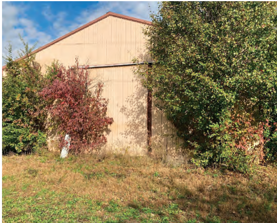
View from the south looking north (Proposed Restroom Location)
