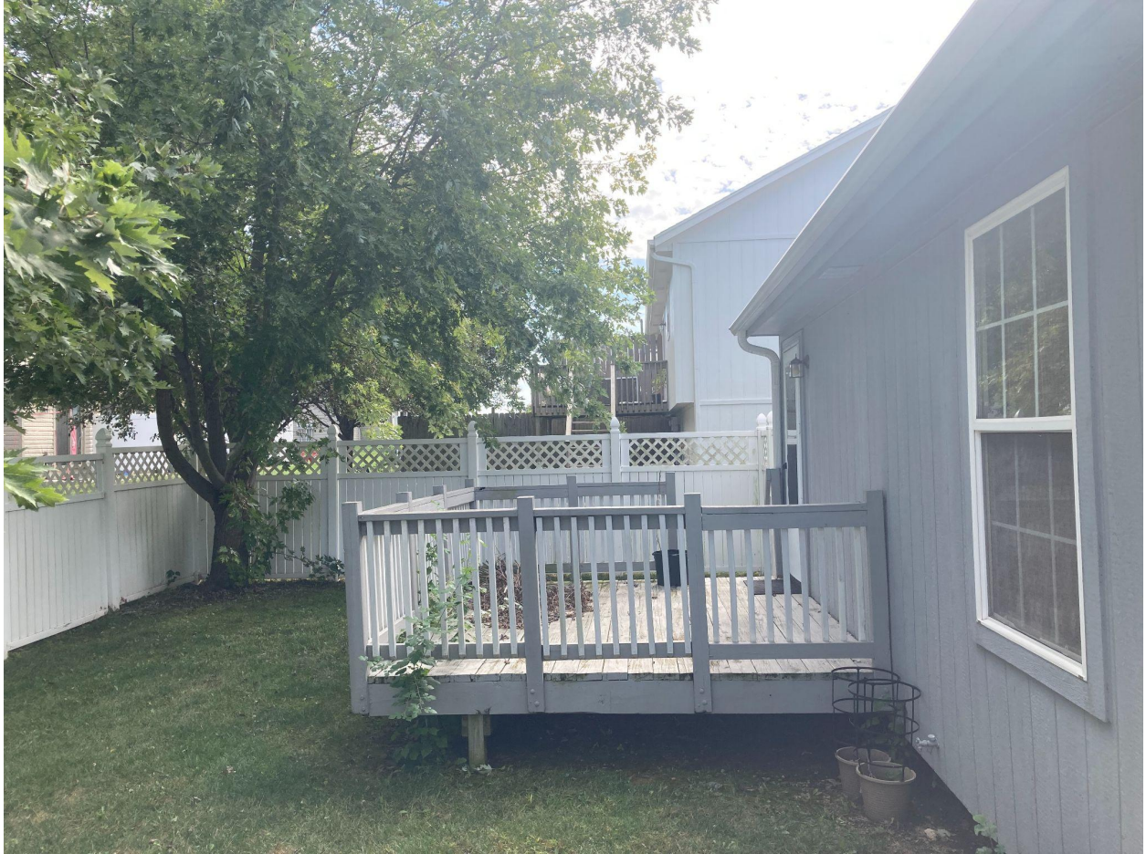
Neighbor to the South with unpermitted uncovered deck
