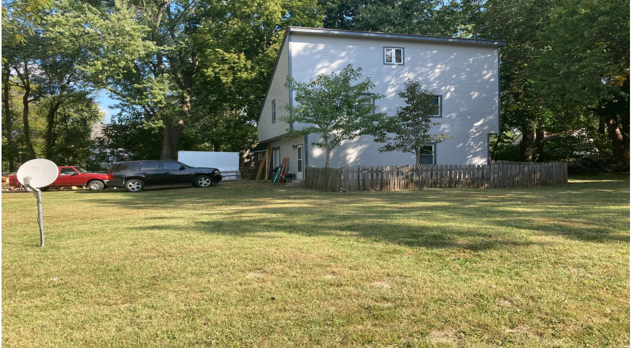
View Looking North from W. Elm St.
