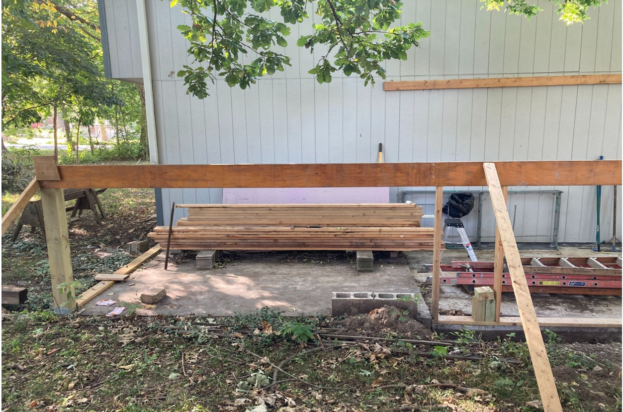
View looking South from North Property Line
