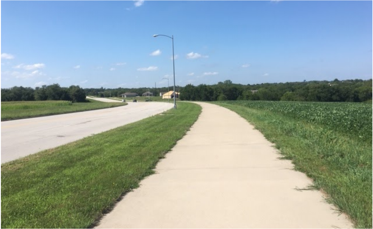
View looking north along Dean Avenue, located roughly at the proposed subdivision entrance.
