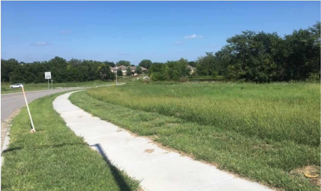
View looking east along Fox Ridge Drive towards the Wood Creek and Stonegate Subdivisions.
