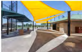
Sun shades at the Recreation Park baseball complex.
