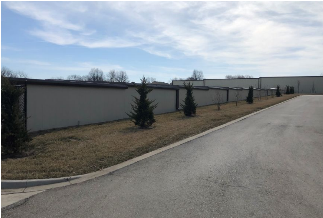
Back of Wall Screening on West Side:
