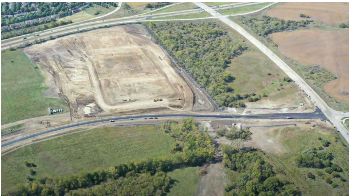
Aerial view looking from the east to the west.
