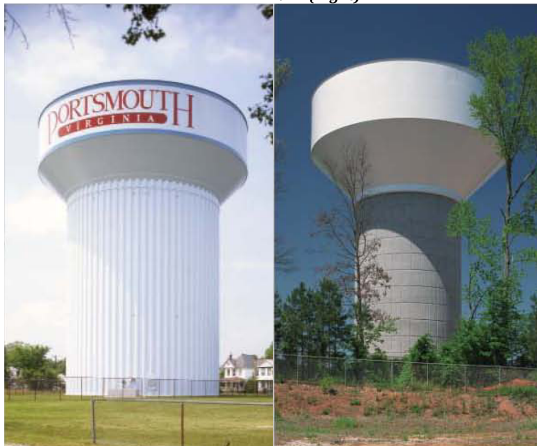
Figure 7-2, Examples of a Fluted Column Elevated Tank (left) and Composite Elevated Tank (Right)
