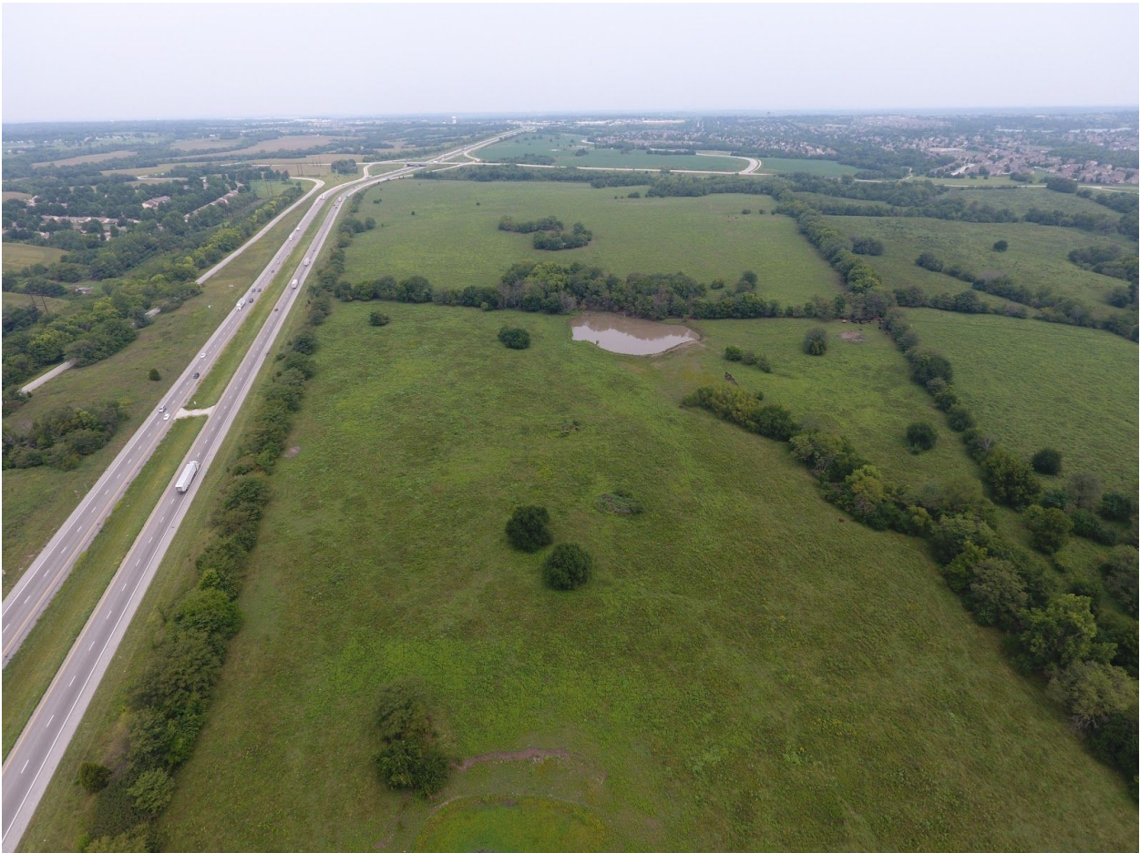
Aerial View looking north toward N. Cass Parkway from the southern property line.
