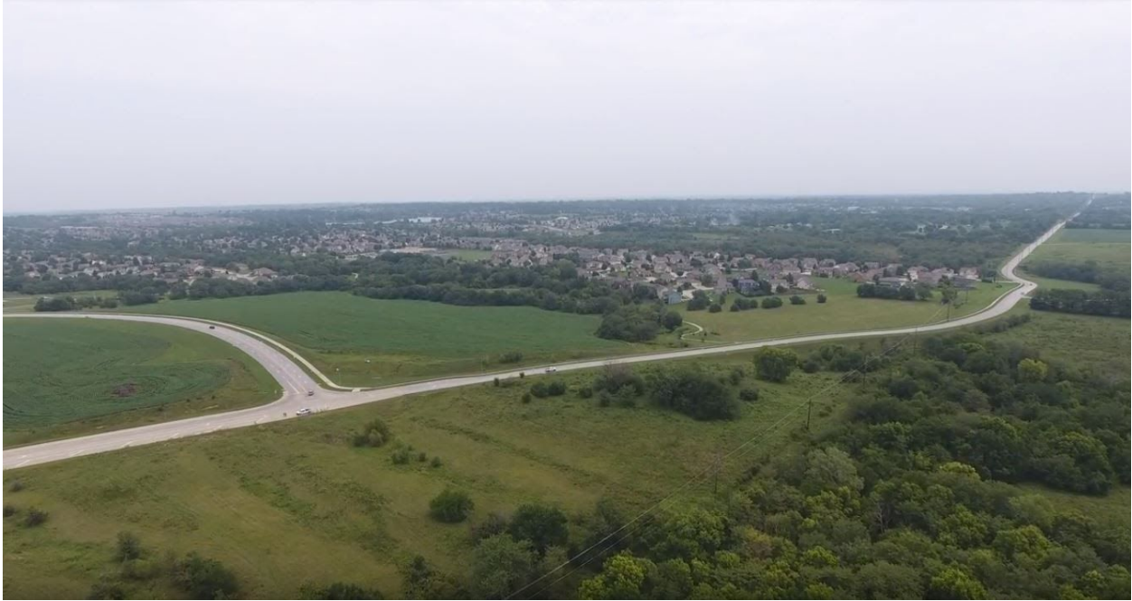
Aerial view looking northeast at Dean Avenue and North Cass Parkway.
