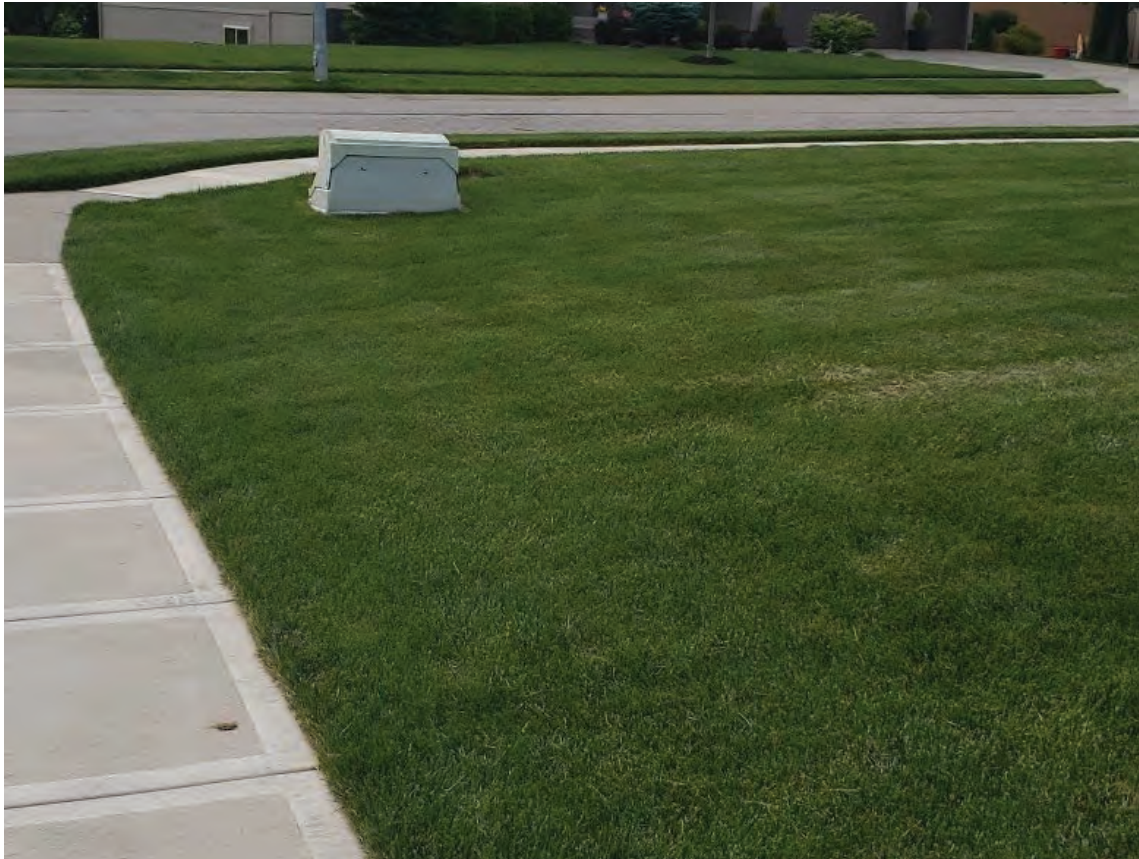
View looking northwest from the southern property line showing the location of the existing utility box in the front yard
