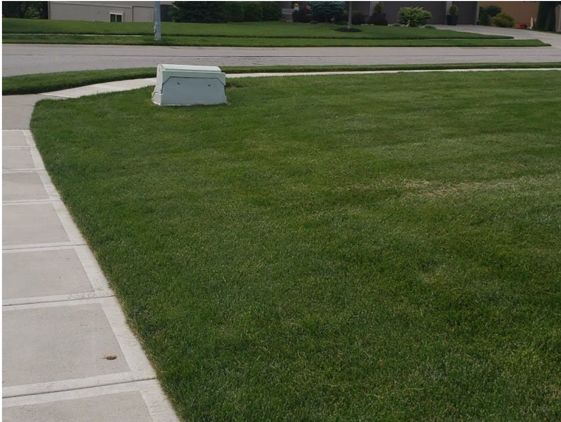
View looking northwest from the southern property line showing the location of the existing utility box in the front yard
