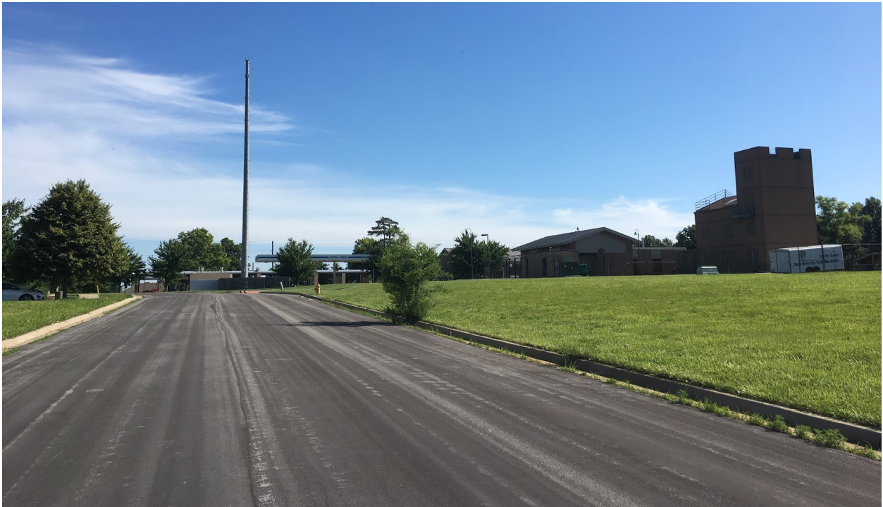
View looking north along Conway Street at the South Metro Fire Station near the project's north property line.
