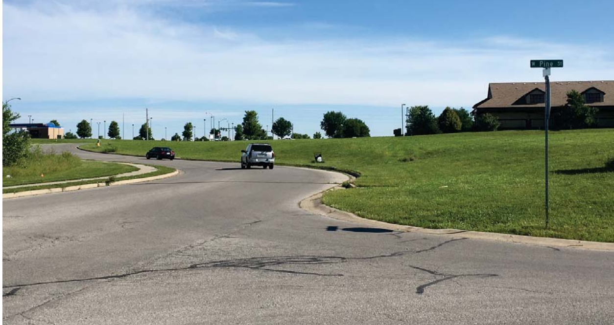
View looking north along Sunset Land from the intersection of Sunset and W. Pine.
