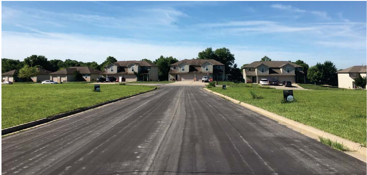
View looking south along Conway Street toward the existing two-family dwellings along W. Pine Street.
