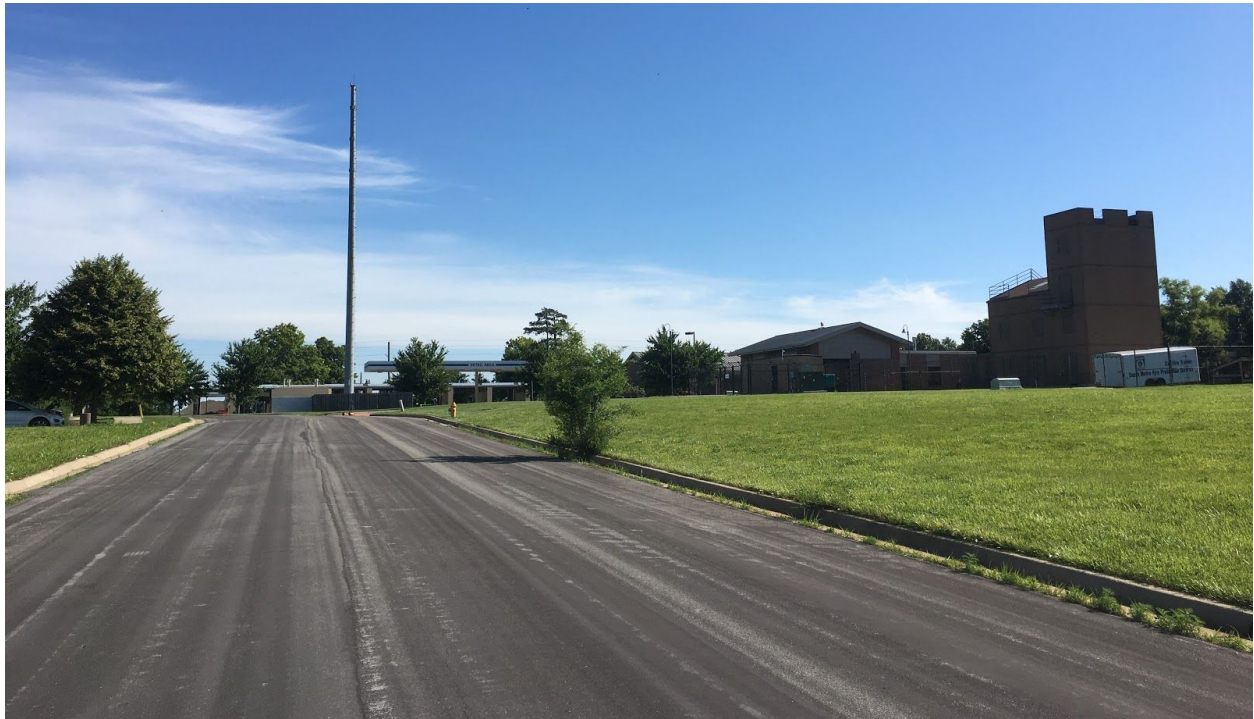
View looking north along Conway Street at the South Metro Fire Station near the project's north property line.
