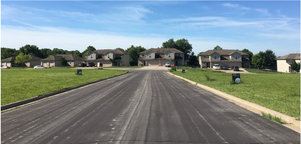
View looking south along Conway Street toward the existing two-family dwellings along W. Pine Street.
