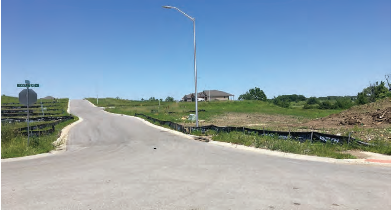
View looking north along Bridgeshire Drive toward Edgewater 6th Plat.
