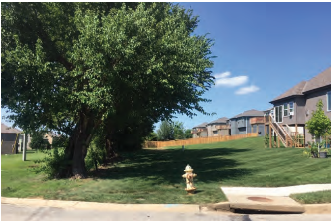
View looking at the north side of Hampton Drive at Lot 166 (614 Laurus Drive).
