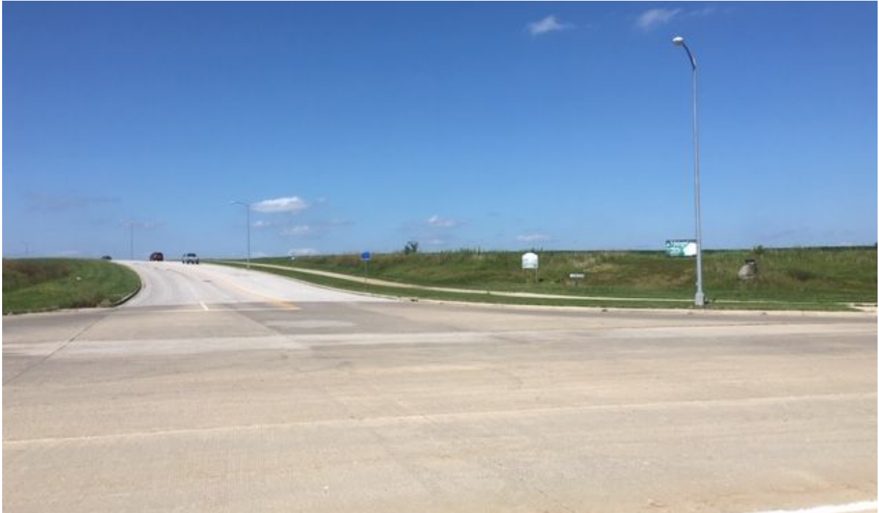
View looking north along Dean Avenue from the southeast corner of the proposed site.
