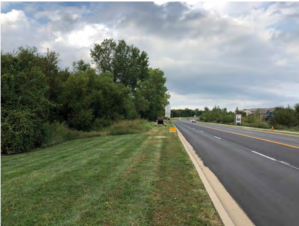
View looking north from the south property line
